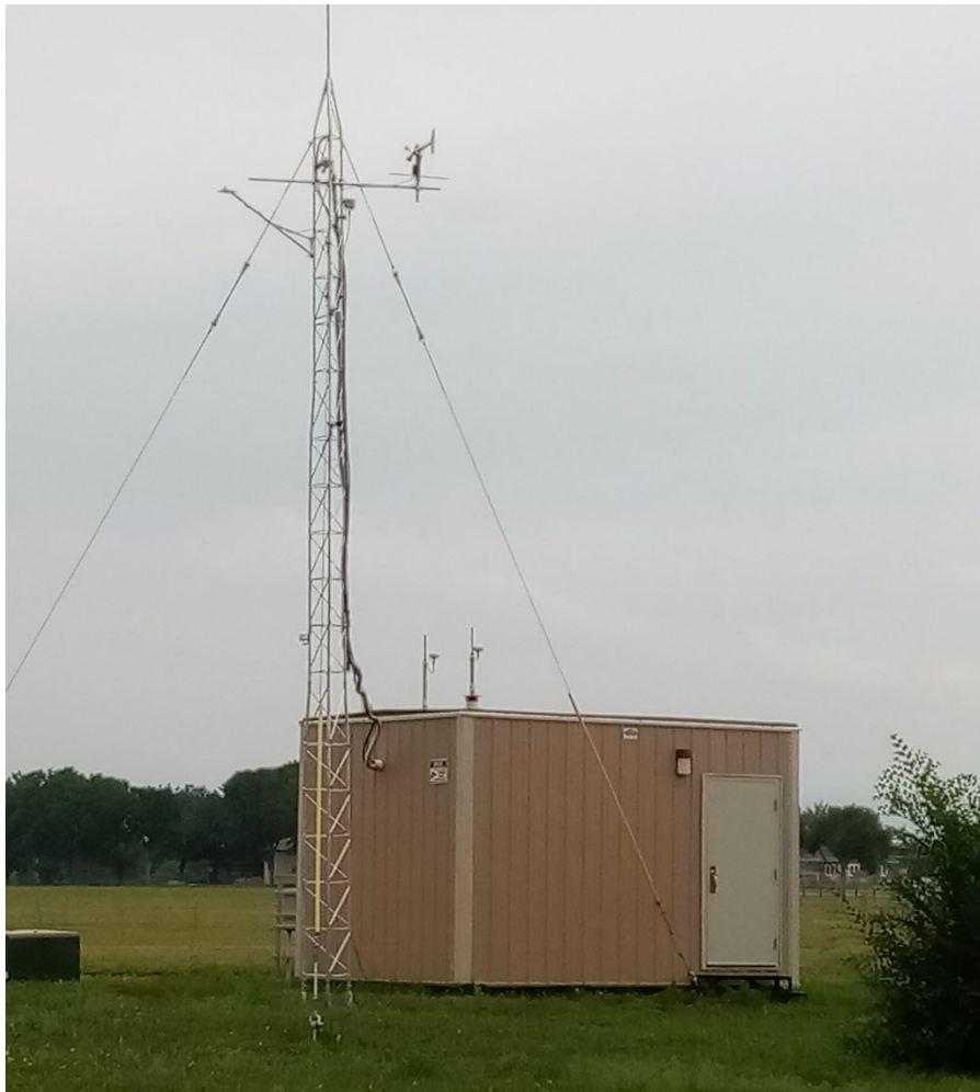
Longmont Union Reservoir (LUR) during summer 2022. The two roof inlets for the intercomparison of the two GRIMM Particulate Matter instruments can be seen side-by-side on the south side of the building.
