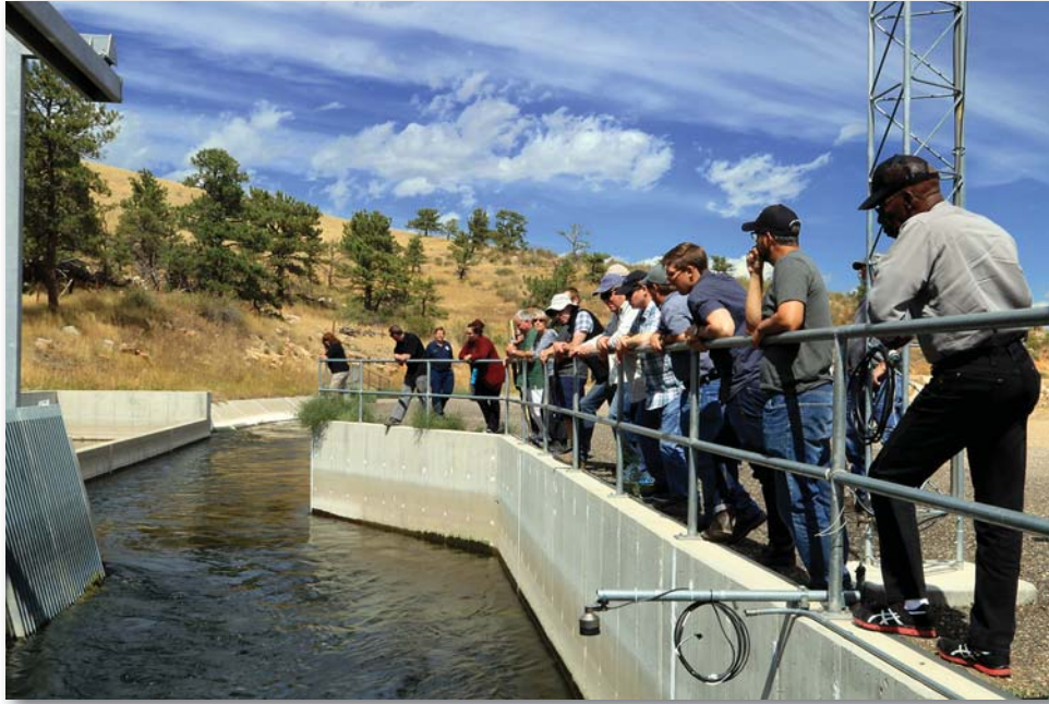
The St. Vrain Supply Canal delivers water from Carter Lake to the Little Thompson River, St. Vrain Creek and Boulder Creek and Reservoir.
