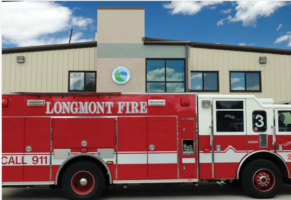
Longmont fire truck at newly remodeled Fleet Services facility
